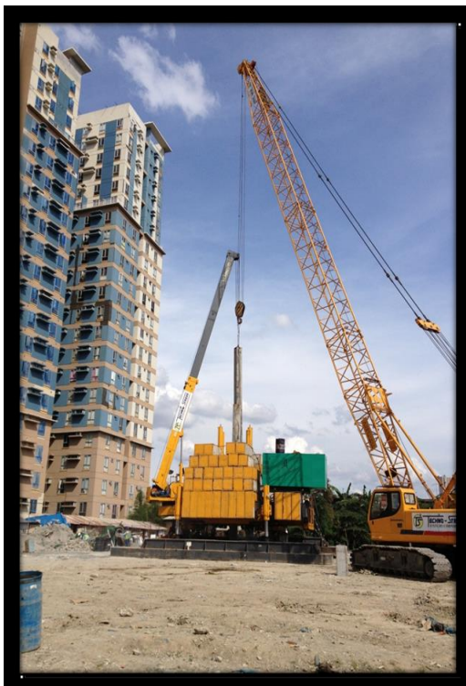
STATIC PILE DRIVER (PUSHED PILE)
